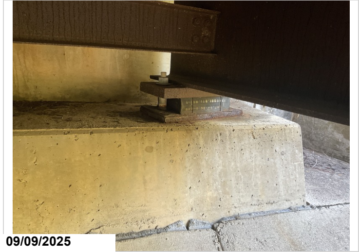
Bent 4, bearing 6, masonry plate has laminating rust. 1EA CS3 Common all bearings at bents 1&4.
