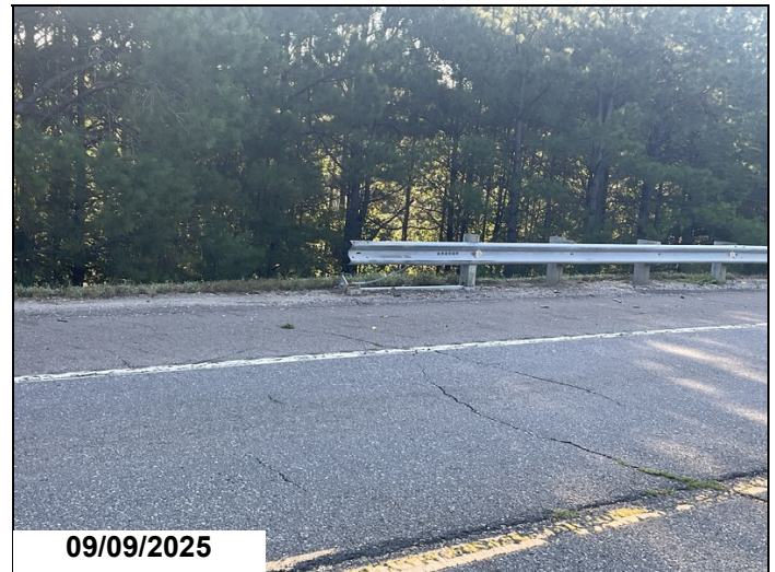
Northeast guardrail damaged from traffic impact.
