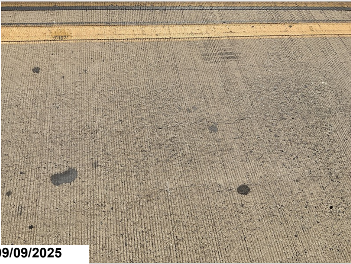
Longitudinal cracks in the deck 0.040". 10SF CS2
