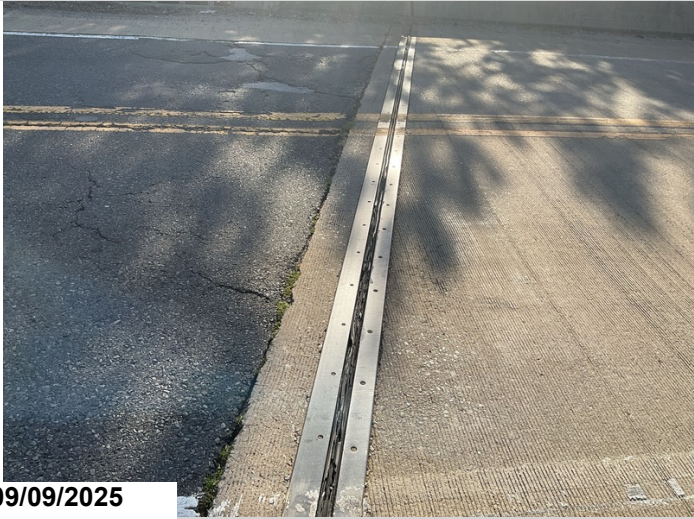
Bent 1 southbound lane joint seal is damaged. 22LF CS2
