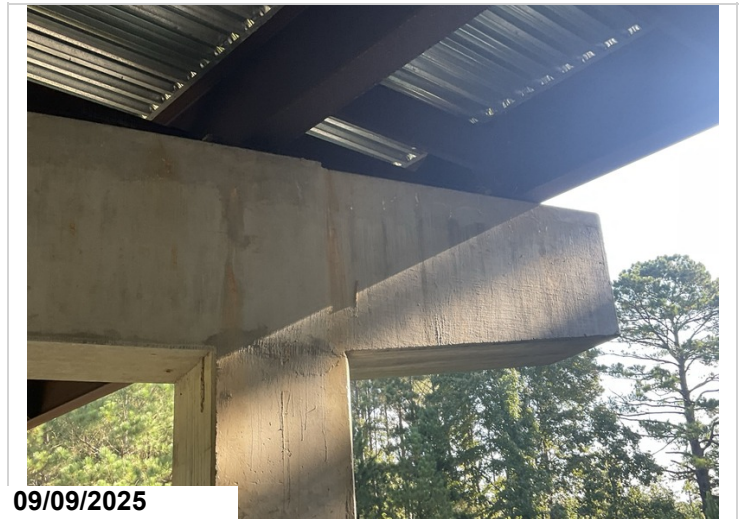
Bent 3 ahead left side cracks with efflorescence. 12LF CS2
