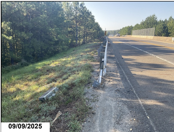
Northeast guardrail damaged from traffic impact.
