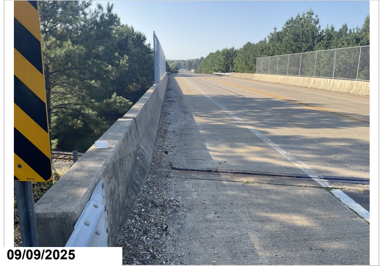
Debris has accumulated on both shoulders.
