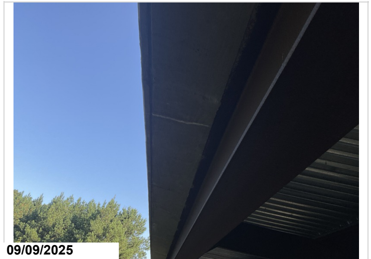
Span 3 right overhang crack with efflorescence. 1SF CS2
