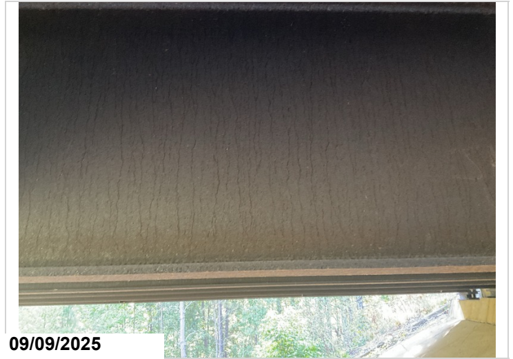
Typical condition for all girders. All girders have a granular texture.
